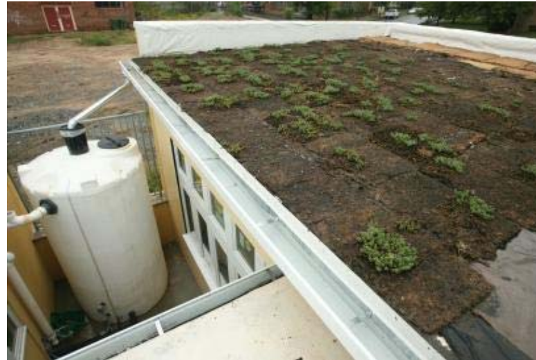
A 2,820-square-foot building on Edgewood Avenue, the first LEED platinum building in Atlanta, has a green roof, and a cistern that captures rainwater.
